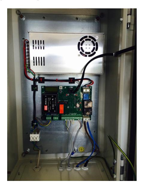
In the control box is the transformer placed above. Maximum output is 12 amp with 24 Volt DC. The maximum effect is therefore 288 Watt.
